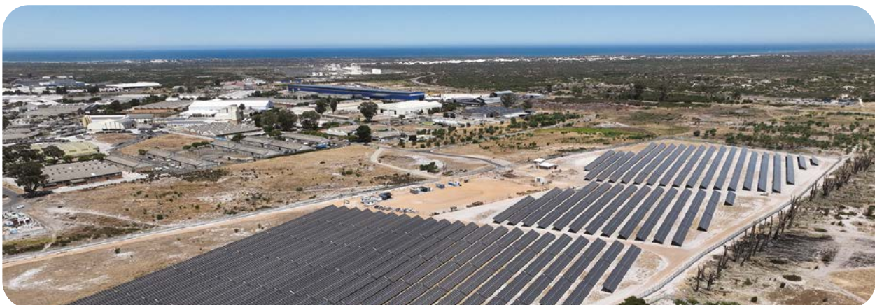
Construction of the City's Atlantis 7 MW solar PV facility was well under way at the time of reporting.
