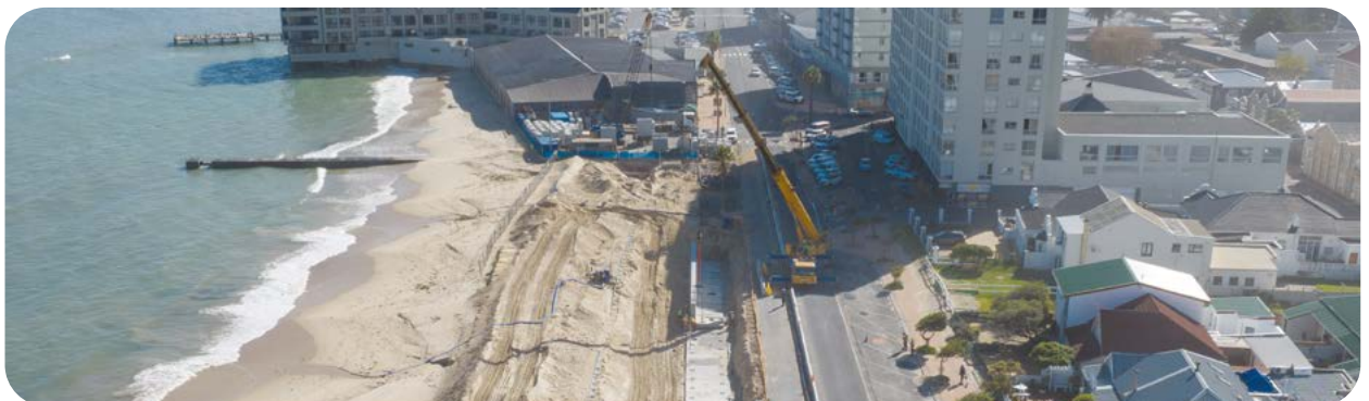
Work on the upgrade of coastal infrastructure is under way, including the sea wall at Strand.
