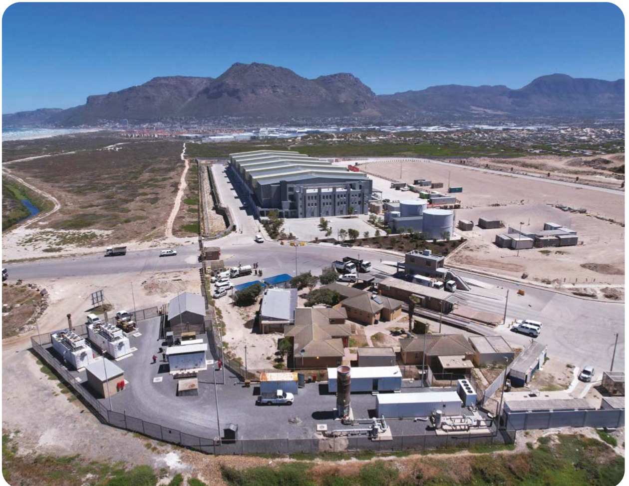
Coastal Park Material Recovery Facility and landfill gas-to-energy plant in progress.
