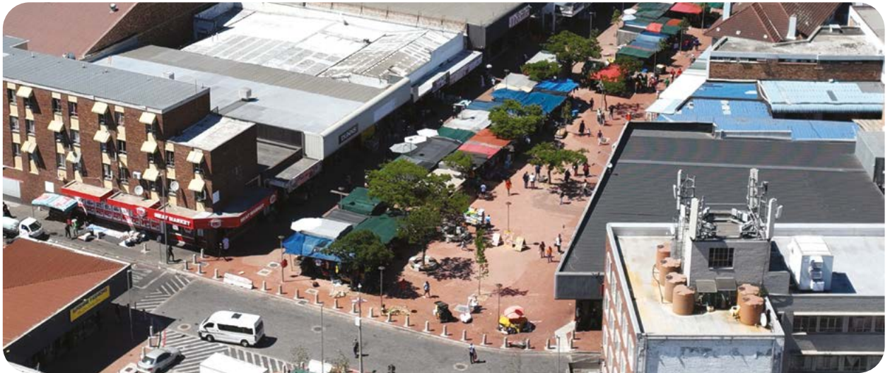
Urban infrastructure improvement projects such as the Kruskal Avenue upgrade project in Bellville was under way during reporting year.
